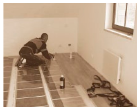
ECOFILM F connection in parallel with Mastic
