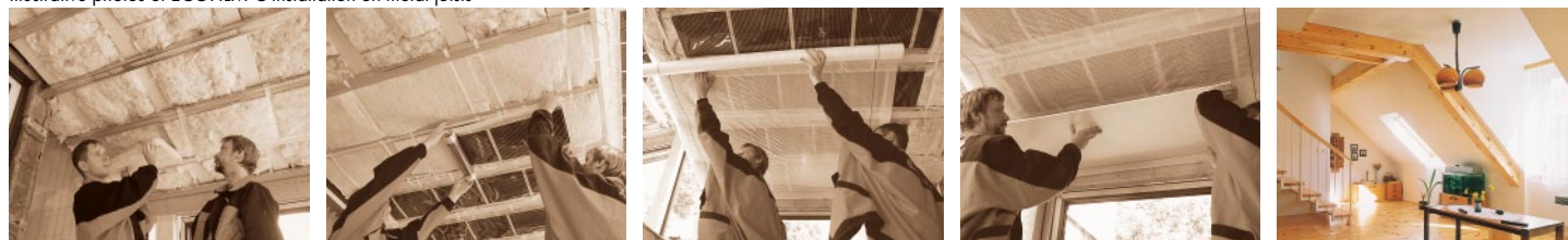
Illustrative photos of ECOFILM C installation on metal joists
